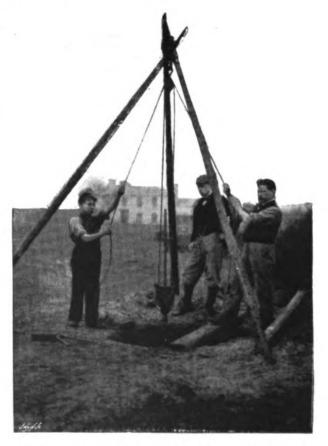
No. 8.—Driving an Abyssinian tube at Pembrey (Wales) to get the water at the spot and at the depth indicated by a diviner. From a photograph by M1. A. E. Lane, Llanelly.
